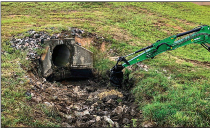
Big-box out flow culvert pipe is damaged from years of high capacity storm water run off.
