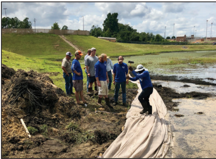
The SOX material is laid out and the staking system is pounded in place.
